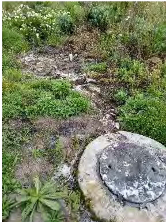
Figure 6. Typical spill from sewer a manhole.
